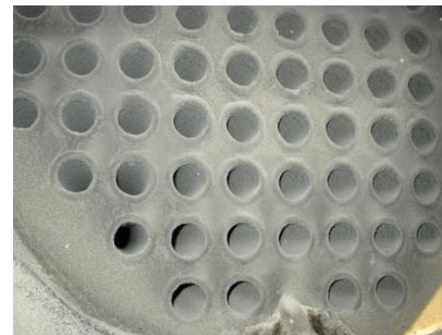
Figure 4-19: Fire-tube boiler (opened) [75]
